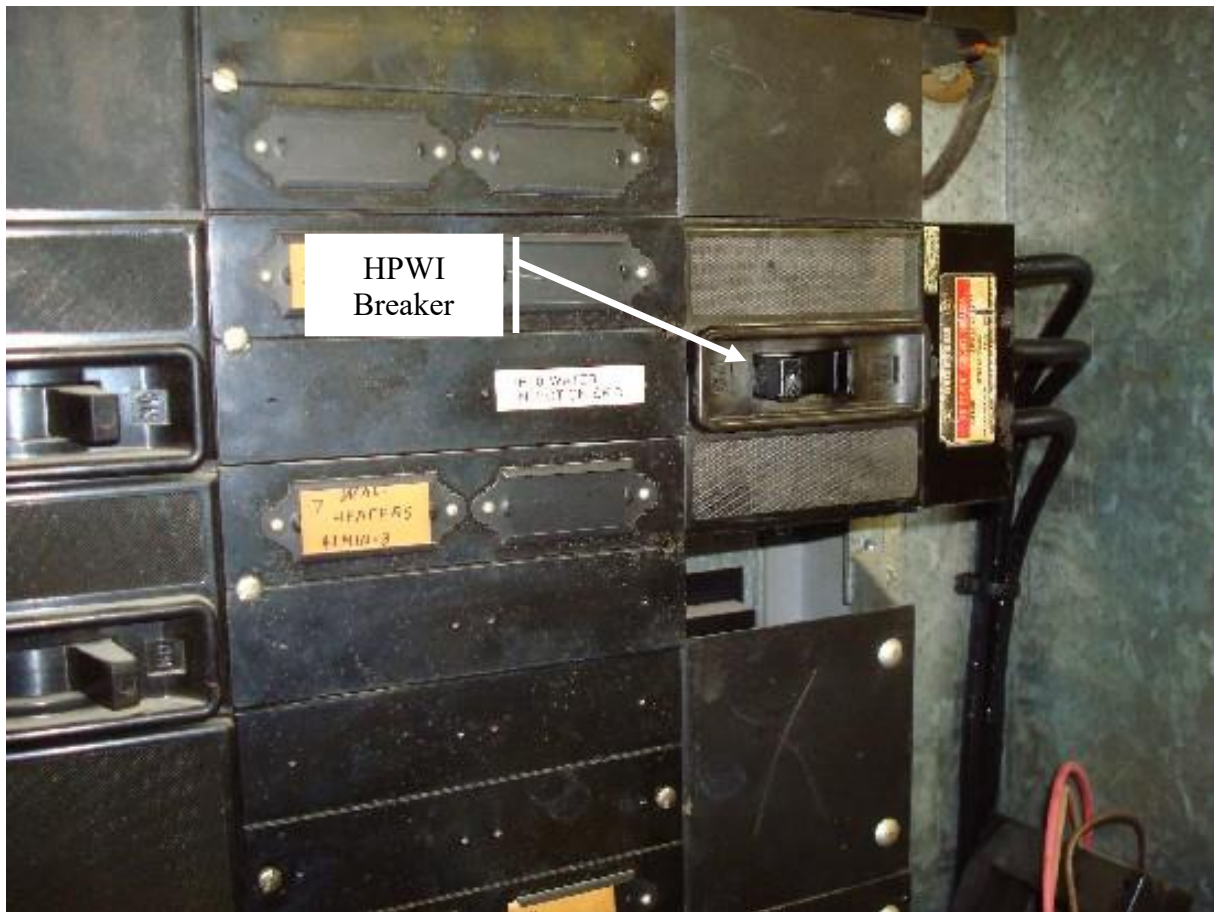
Figure 14 – 480 volt supply breaker
