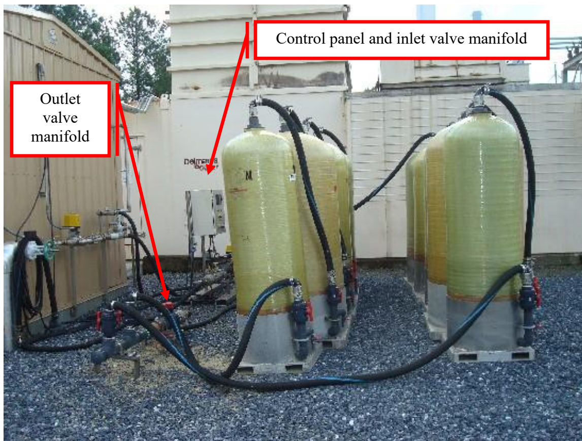
Figure 12 - Demineralizers
