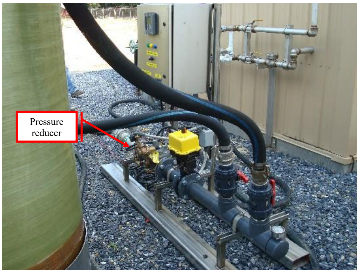
Figure 13 – Demineralizer inlet and control panel
