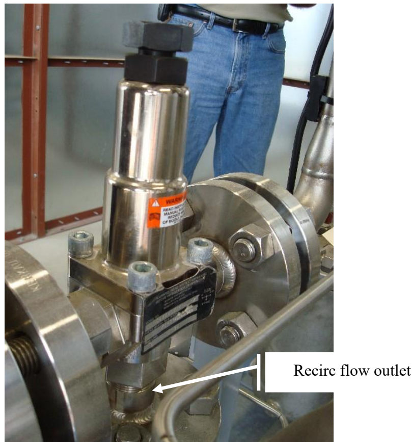
Figure 9 – Pressure control recirculation valve
