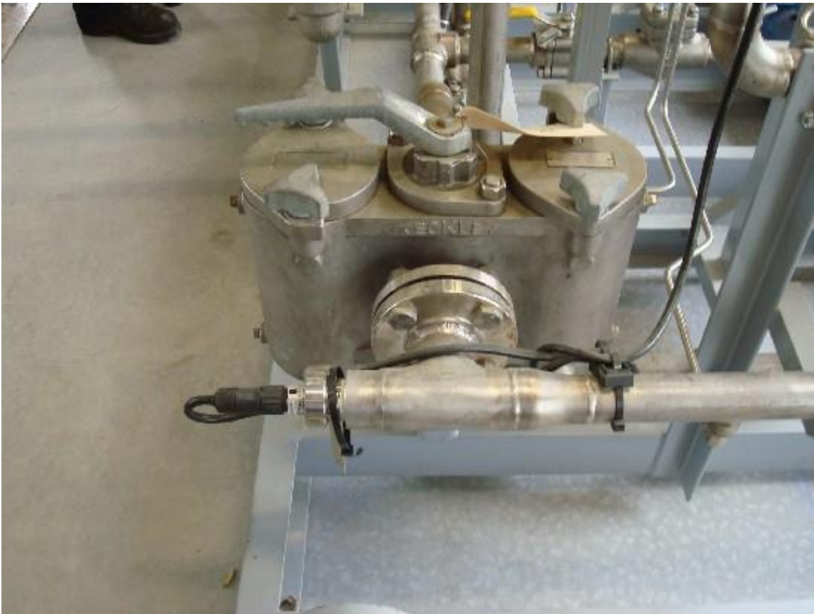
Figure 6 – Duplex strainer
