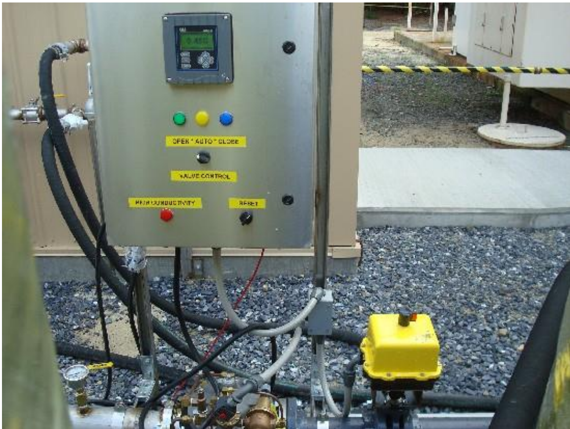
Figure 18 – Demineralizer control panel
