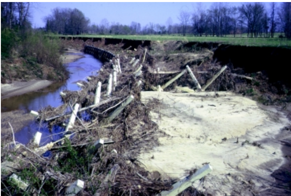
Figure 16-31 Concrete jack system several years after installation
