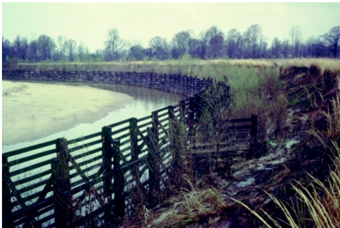
Figure 16-28 Slotted board fence system
