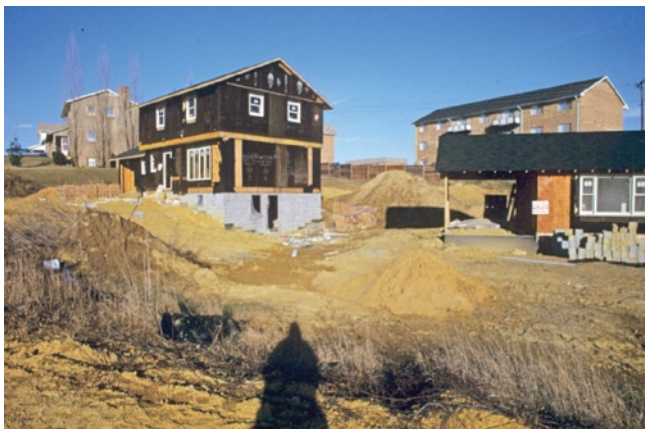
Figure 3.2. Typical soil disturbance in subdivision during construction. Each lot is graded out (cut and filled) to approximately level the area immediately surrounding the house. Note large amounts of sand and other construction debris that will more than likely be graded out and incorporated into fills.
