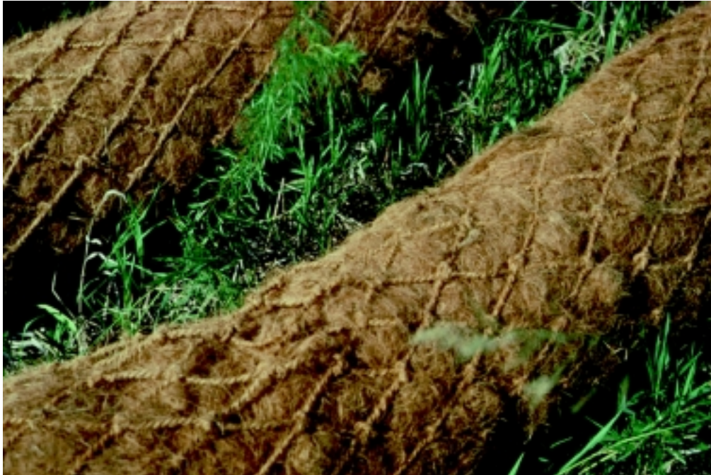
Figure 16-37a Coconut fiber roll
