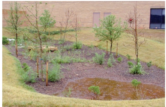
Figure 9.8. Bioretention rain garden.
