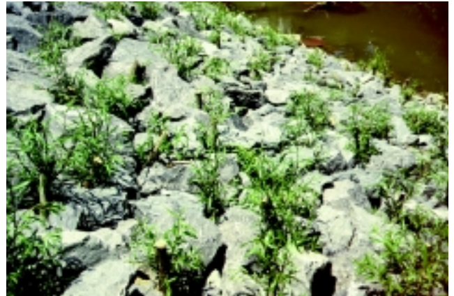
Figure 16-17b An installed joint planting system (Robbin B. Sotir & Associates photo)
