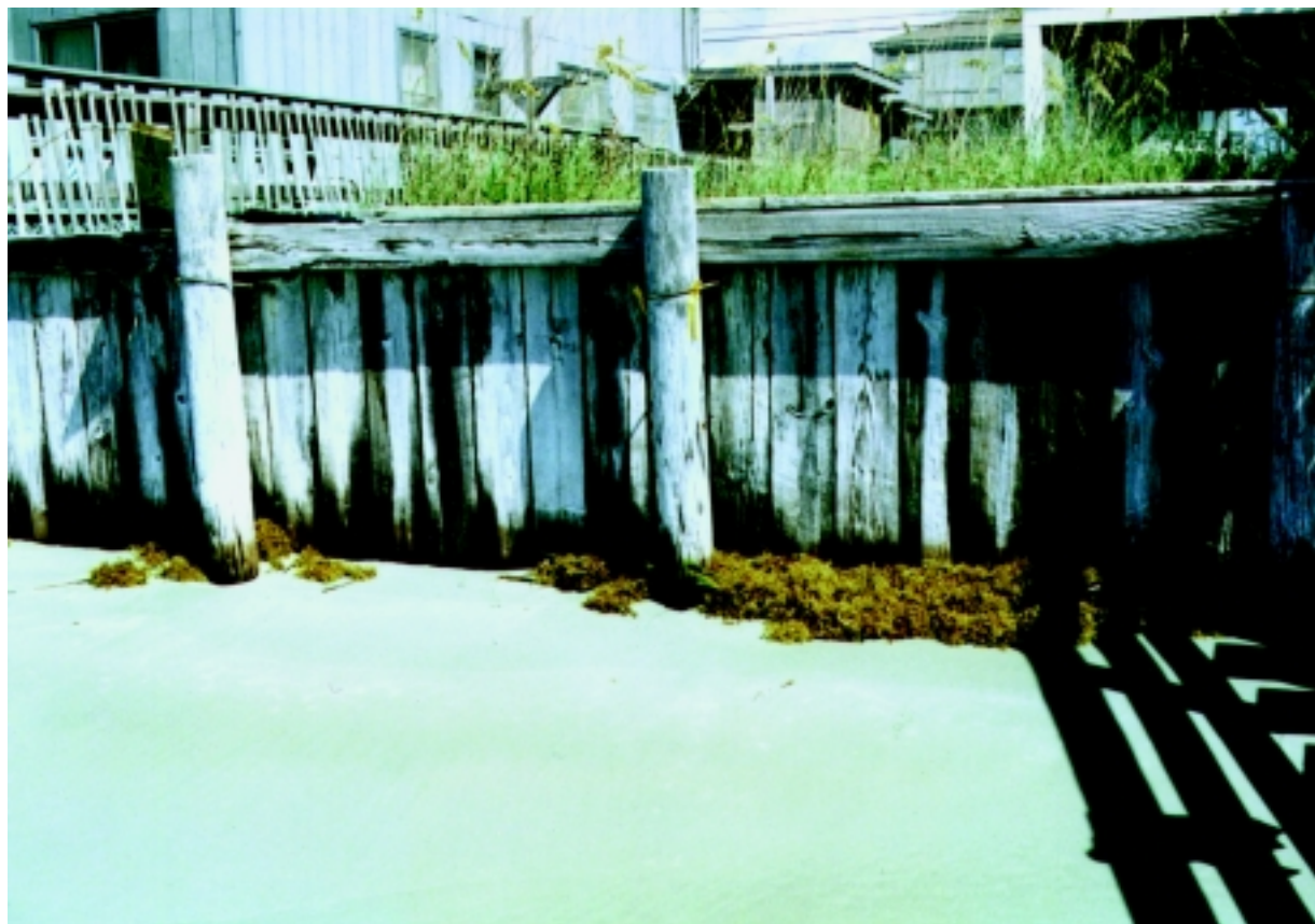
Figure 16-46 Timber bulkhead system
