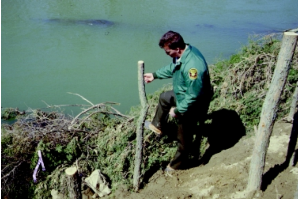
Figure 16-21a Tree revetment system with dormant posts
