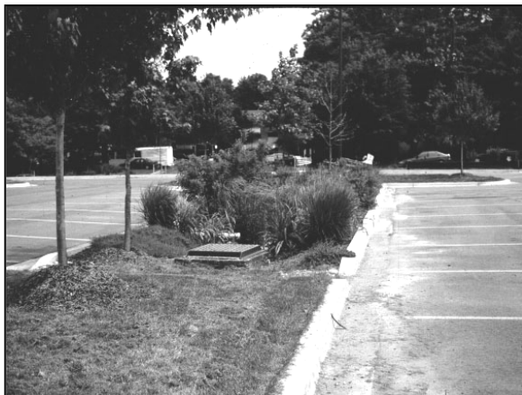
Figure 2: Parking Lot Island Turned Bioretention Area
