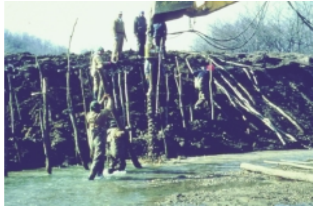
Figure 16-25b Installing dormant posts (Don Roseboom photo)
