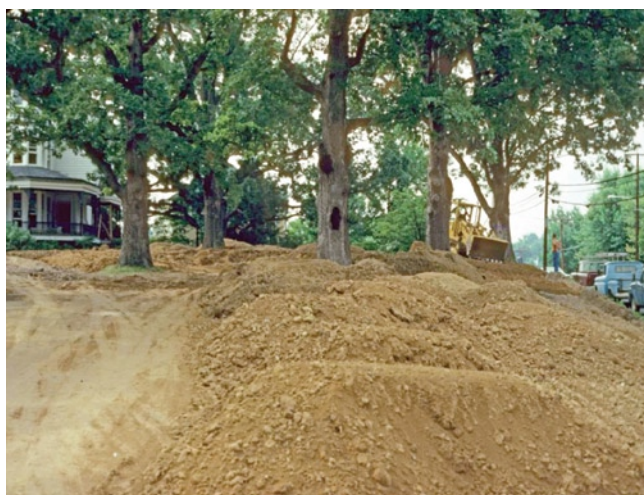
Figure 3.5. Inappropriate addition of topsoil over native trees: The topsoil material was added too thickly (12 inches) and then compacted (as seen at left) to a point that gas exchange by the living tree roots was limited. Most of these white oaks died within two years of this application.
