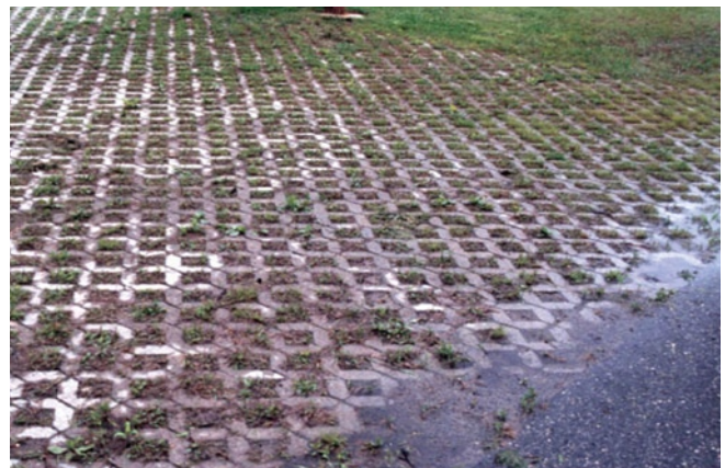
Figure 9.9. Compost can be used as partial growth and filtering medium in pervious pavement.
