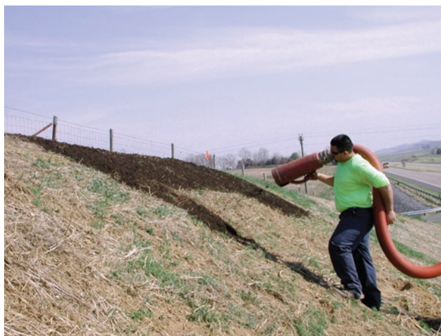
Figure 9.10. Compost applied pneumatically to steep slopes adjacent to highway to establish medium for erosion controlling and hillside stabilizing vegetation. Photo courtesy of Greg Evanylo.
