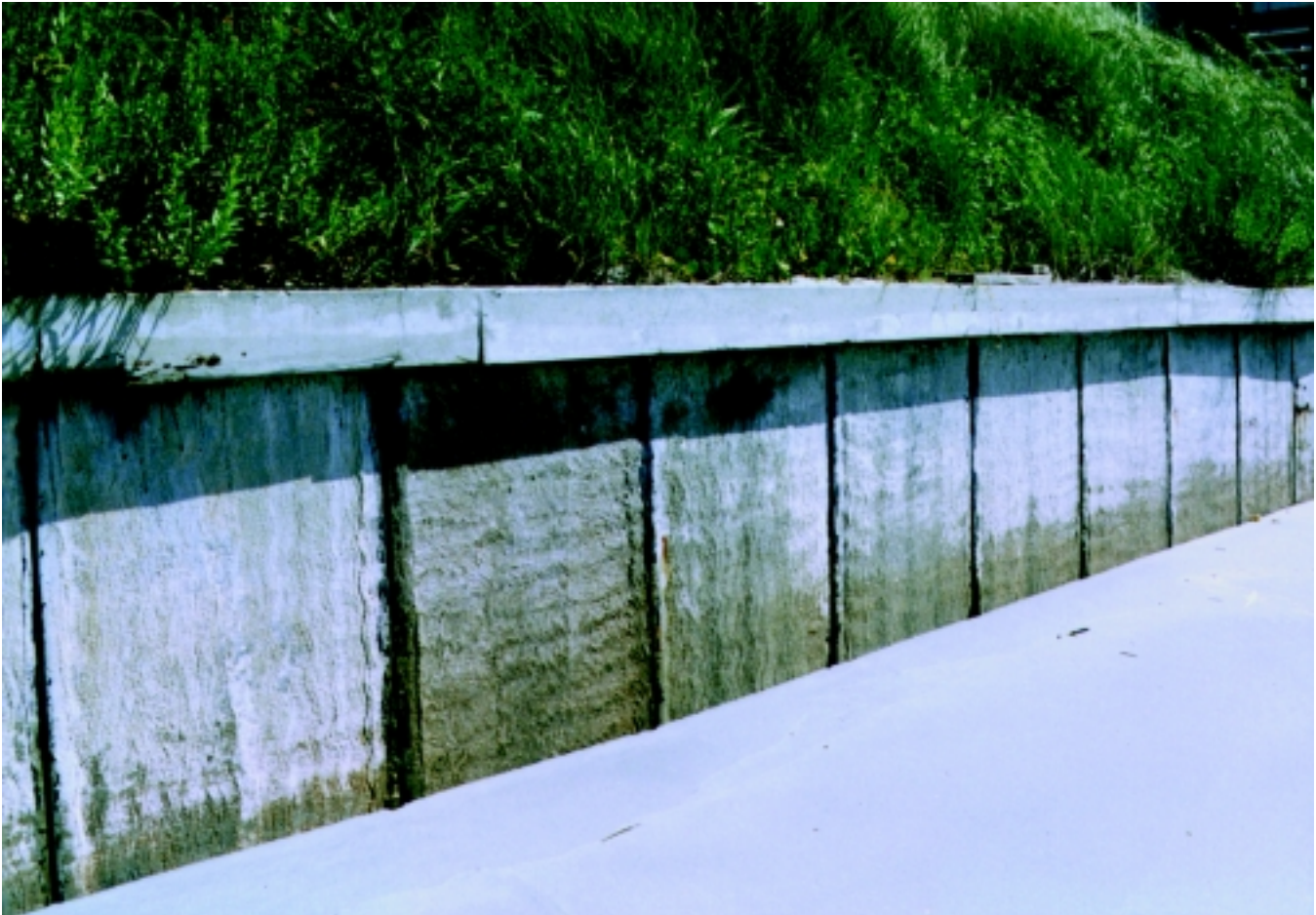
Figure 16-49 Concrete bulkhead system
