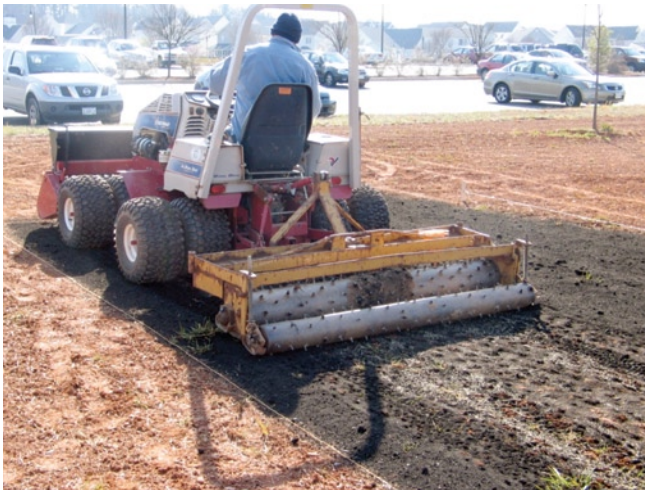
Figure 9.4. Applying turfgrass seed to compost-mulched disturbed soil. Photo courtesy of Greg Evanylo.
