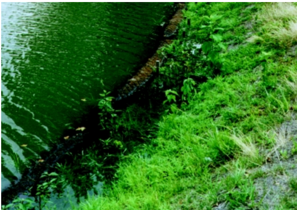
Figure 16-37b Coconut fiber roll system
